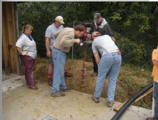
Putting in frame work for new fence at Fall Fellowship
